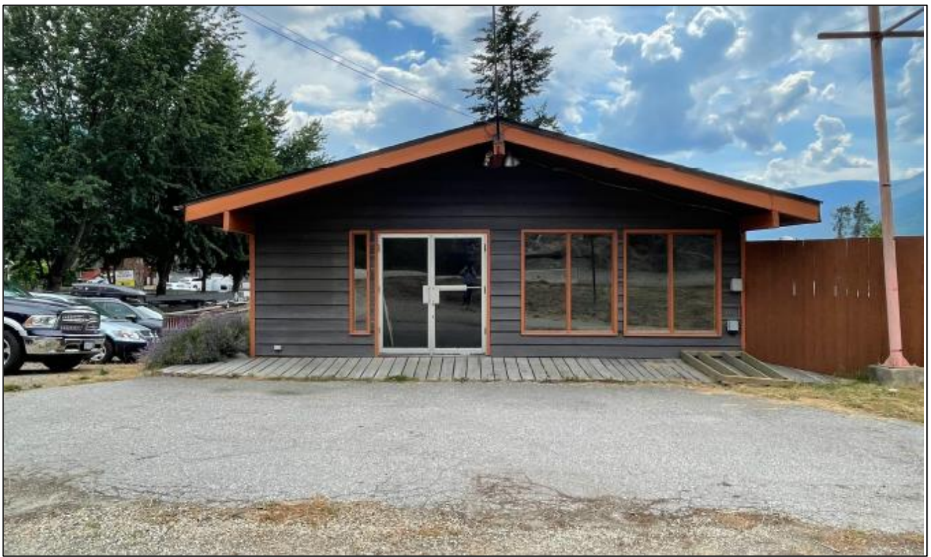
Figure 3: Site Photo of Existing Building (front/eastern elevation)
