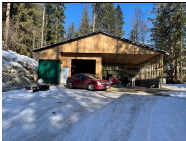
Figure 1: Site Visit Photo of Existing Unauthorized Structure
