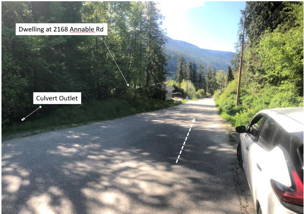
Photo 6: View of looking down (south) Annable Road at creek crossing (600 mm CMP). Culvert blockage during an extreme flood will result in water flowing down the road to the Hwy away from the dwelling on 2168 Annable Road. The road surface gradient is 10%. May 14, 2021
