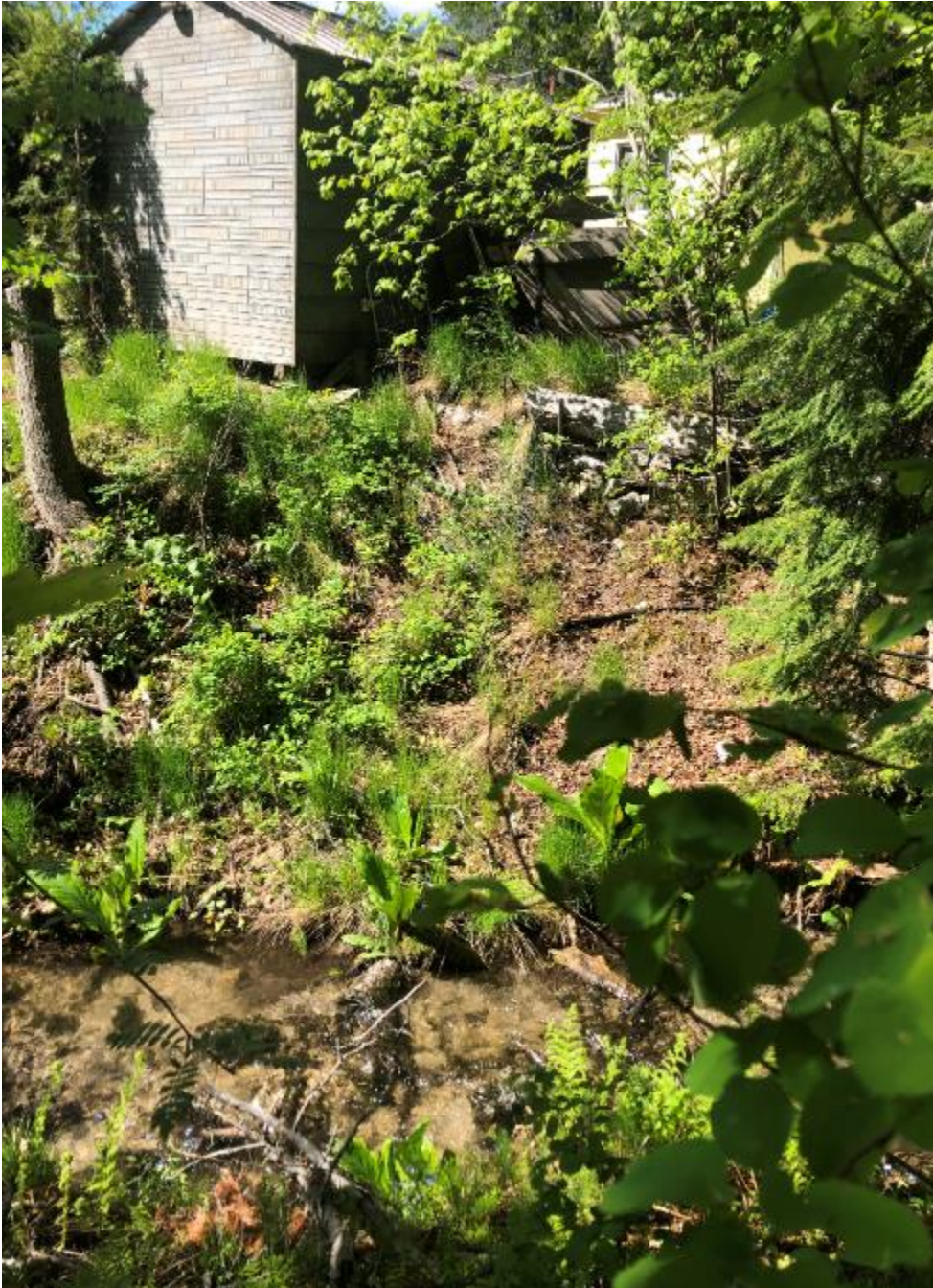
Photo 2: View of Right (south west) Creek Bank and Location of Cross Section Figure 8. Dwelling visible in background behind Shed – May 11, 2021
