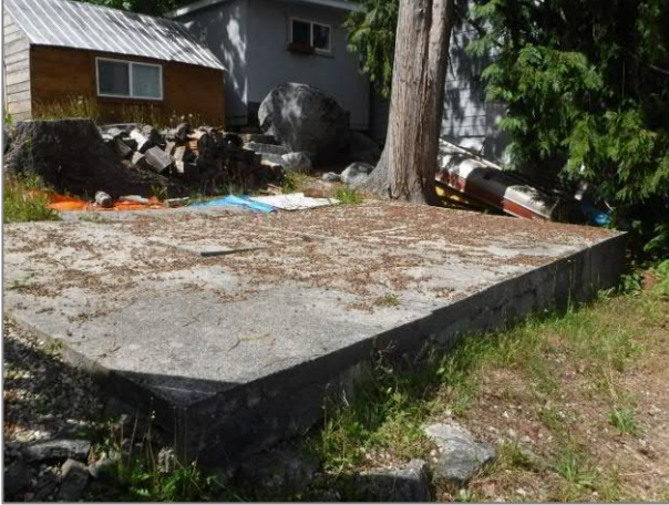
Photo 3. View of concrete slab patio.
