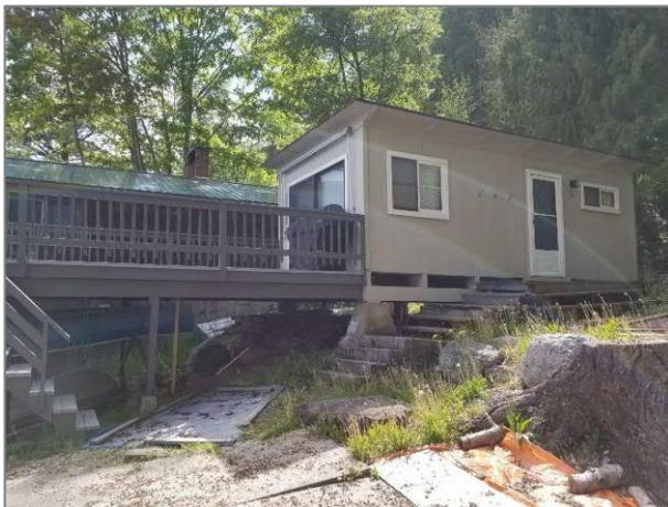
Photo 1. View of existing cabin and raised deck.
