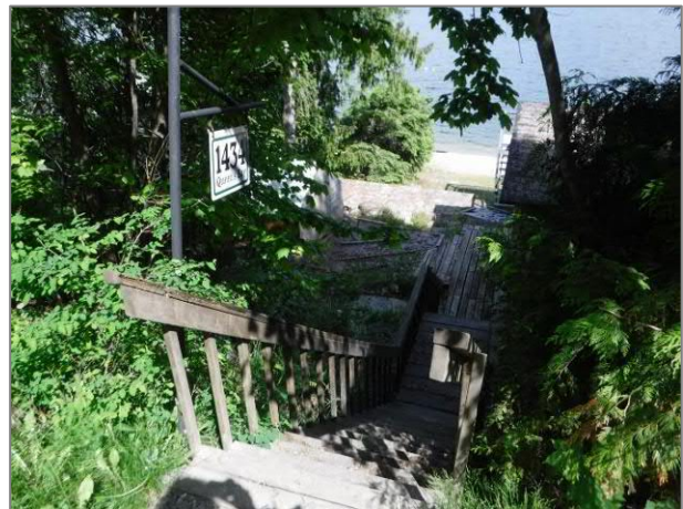
Photo 2. View of highway embankment staircase.
