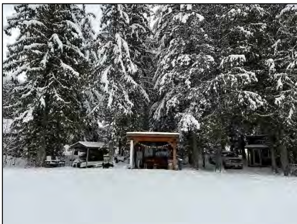
Photo 17. View of boat storage, outdoor kitchen and bunkhouse
