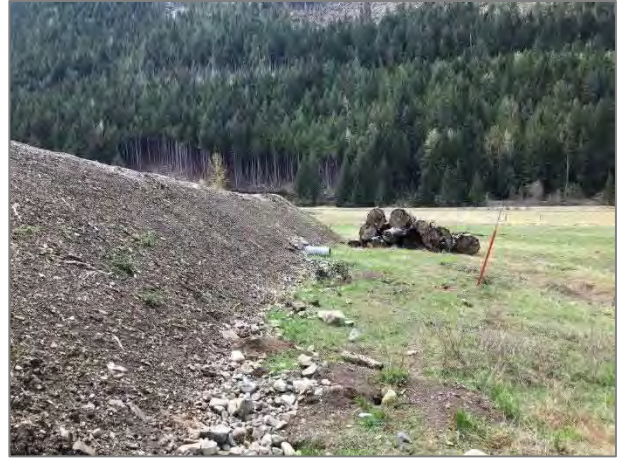
Photo 6. Access road embankment, looking west (May 10, 2023).
