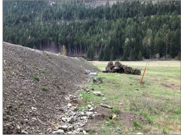
Photo 6. Access road embankment, looking west (May 10, 2023).
