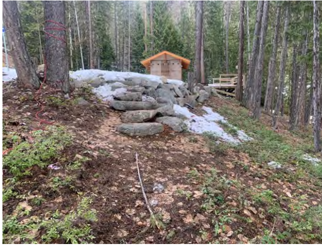
Photo 4 - slope below propert boundary
