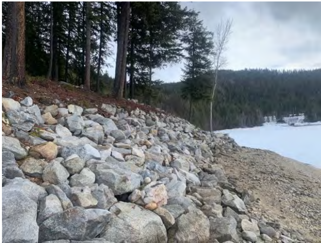
Photo 2 - Shoreline on north end with rip rap
