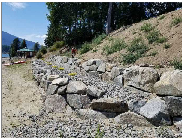
Photo 13. Tiered rock retaining wall. July 27, 2023.
