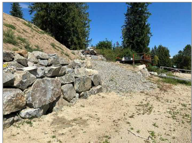
Photo 14. Crushed gravel access road. July 27, 2023
