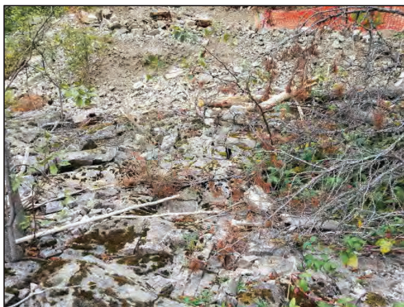
Photo 13. Exposed bedrock along the foreshore fronting the house.
