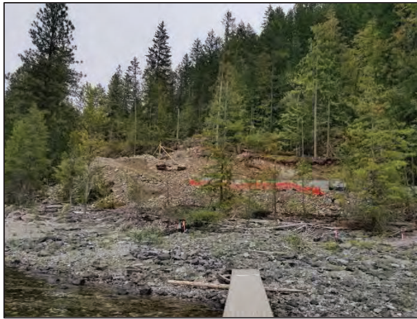
Photo 3. Current view of foreshore disturbance area looking east, Sept 22, 2022.
