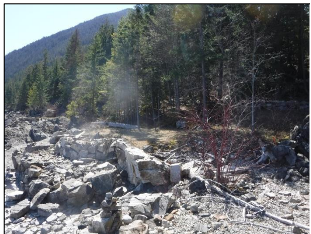
Photo 6. Tiered rock stack retaining walls supporting greenspace terrace.
