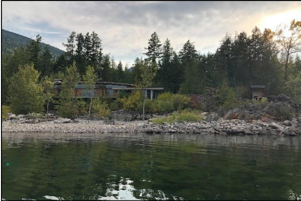
Photo 1. View of existing main house and foreshore area.
