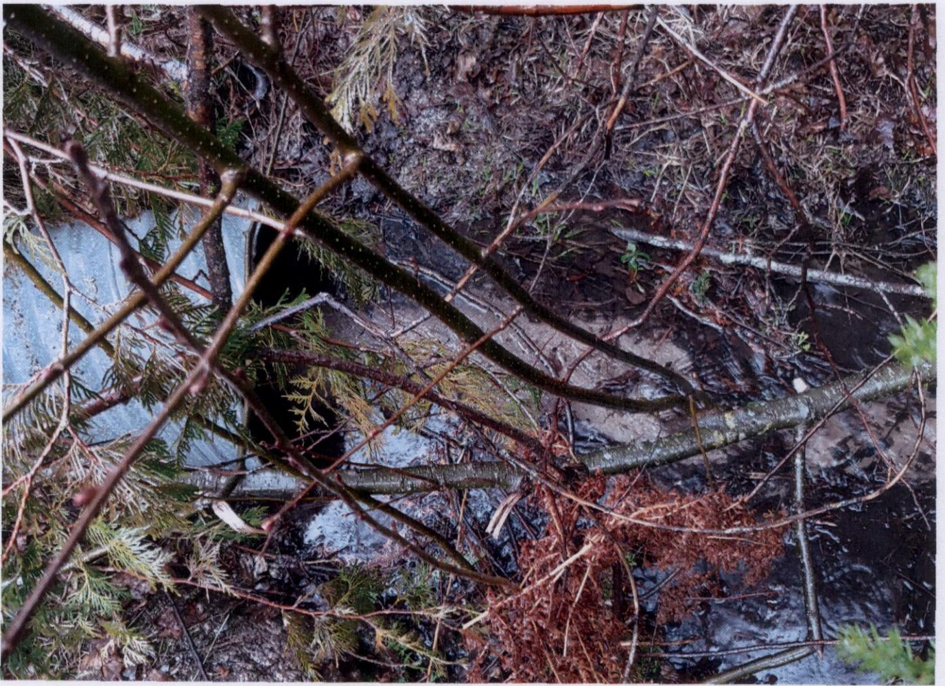
Clear Springs culvert outlet.
