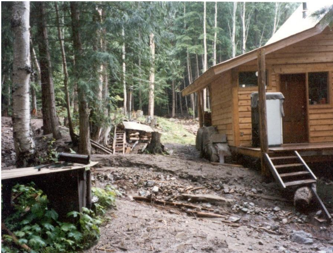
Photo 6 Debris against house after 1990 Slide
