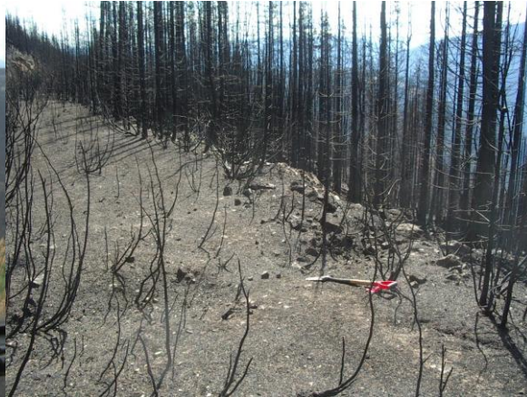
Photo 17 Cross ditch in old road in North Van Tuyl Creek Drainage
