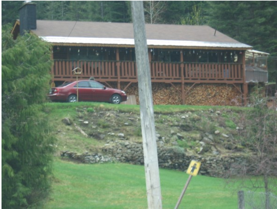
Figure 5. Photograph showing home with open decks and fire wood storage under the home.
