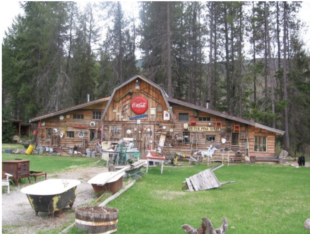
Figure 3. Photograph showing wooden siding present on some homes within the wildland urban interface.
