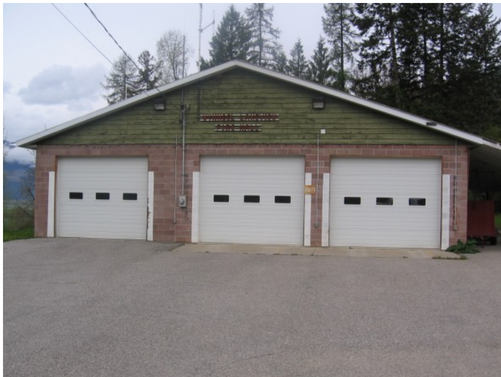
Figure 2. Wynndel-Lakeview Fire Hall.
