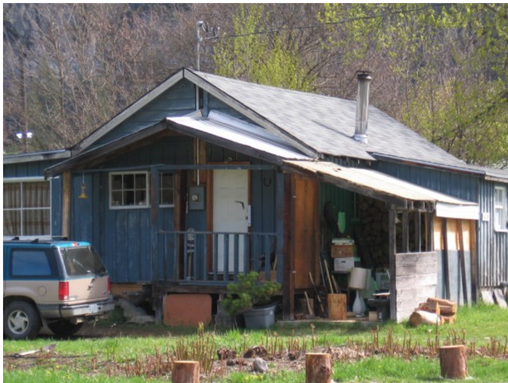
Figure 3. Example of home with wood siding and open decks.
