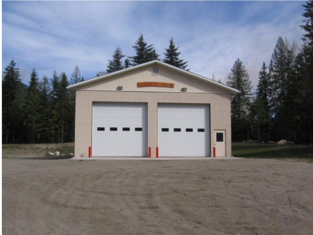
Figure 2. Village of Slocan City Fire Hall.
