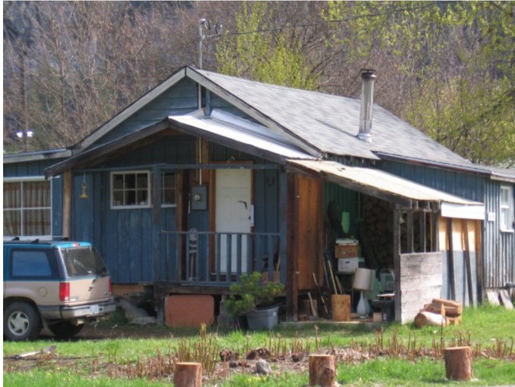
Figure 2. Example of home with wood siding and open decks.
