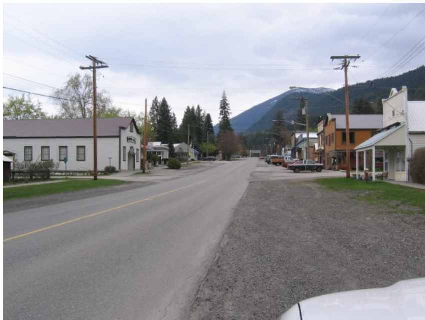
Figure 3. Structures in the main street constructed with fire resistant materials.
