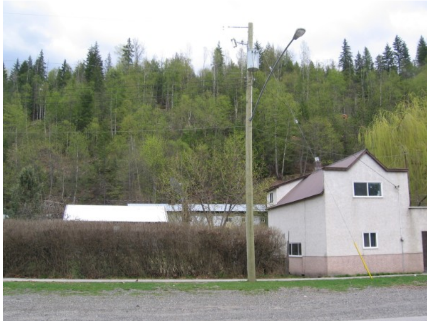
Figure 2. Structure constructed with fire resistant materials.
