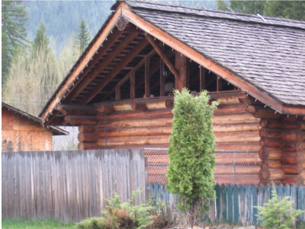
Figure 2. Photograph showing wood shingles and open eaves.
