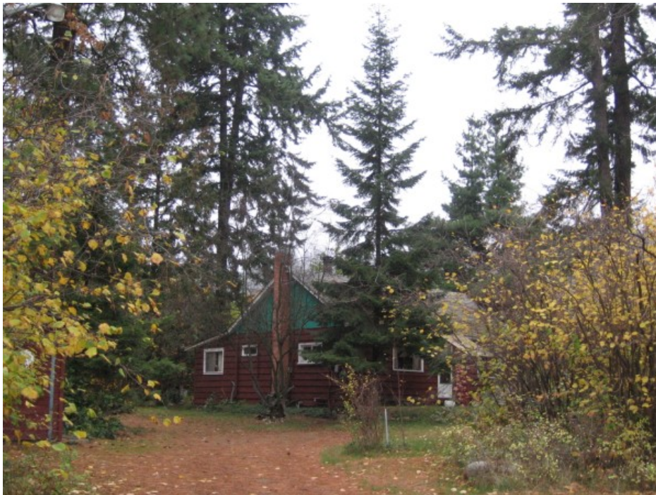
Figure 2. Example of home with wood siding and no setback to forest vegetation.
