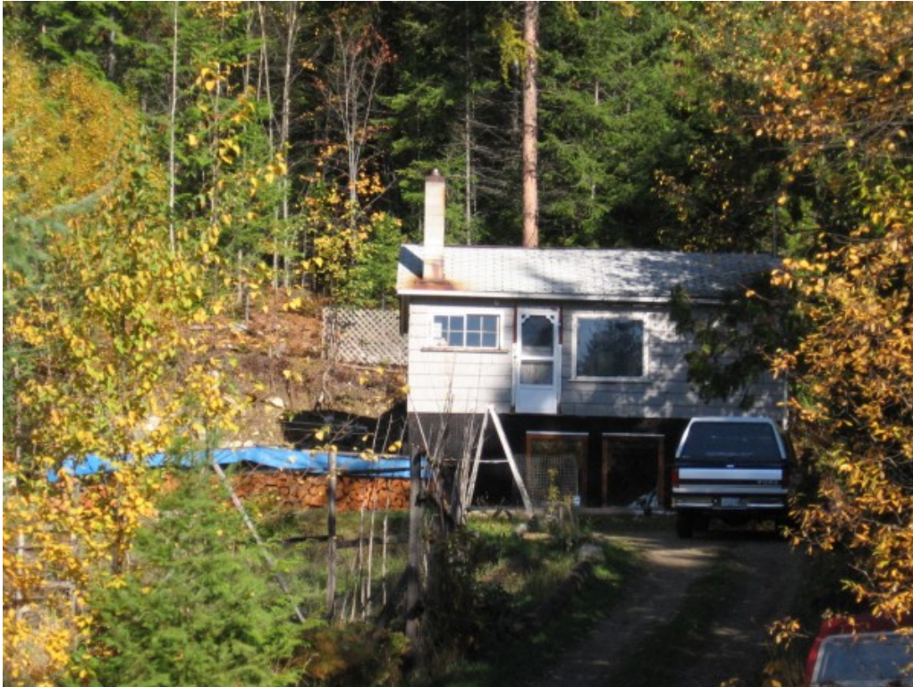
Figure 4. Example of home with firewood adjacent to building and an incomplete setback from forested edges.
