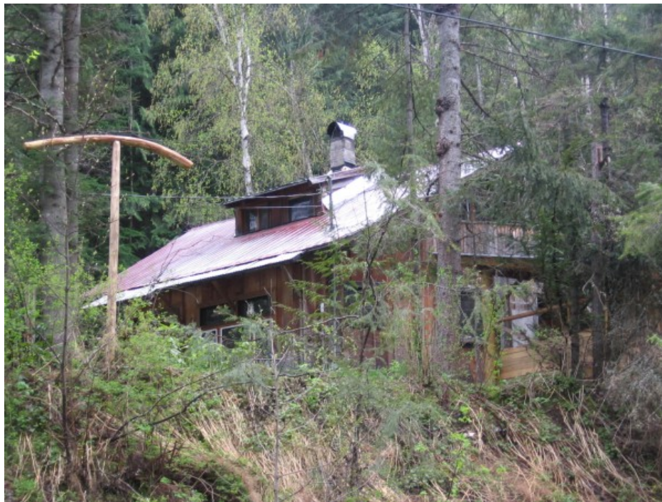
Figure 4. Photograph showing wooden siding and open decks.
