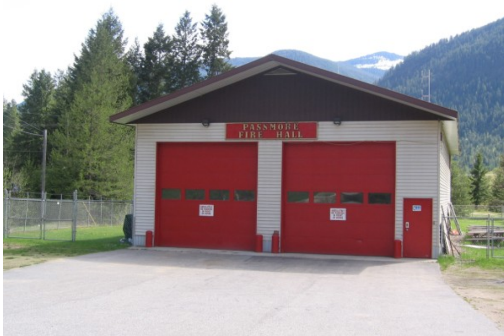
Figure 2. Passmore fire hall.
