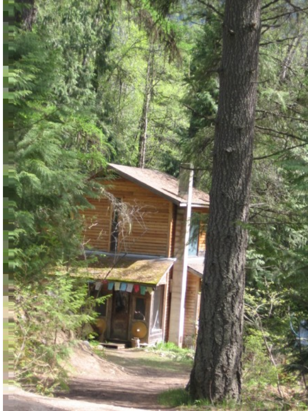
Figure 5. Example of home with wood siding and no setback to forest vegetation.
