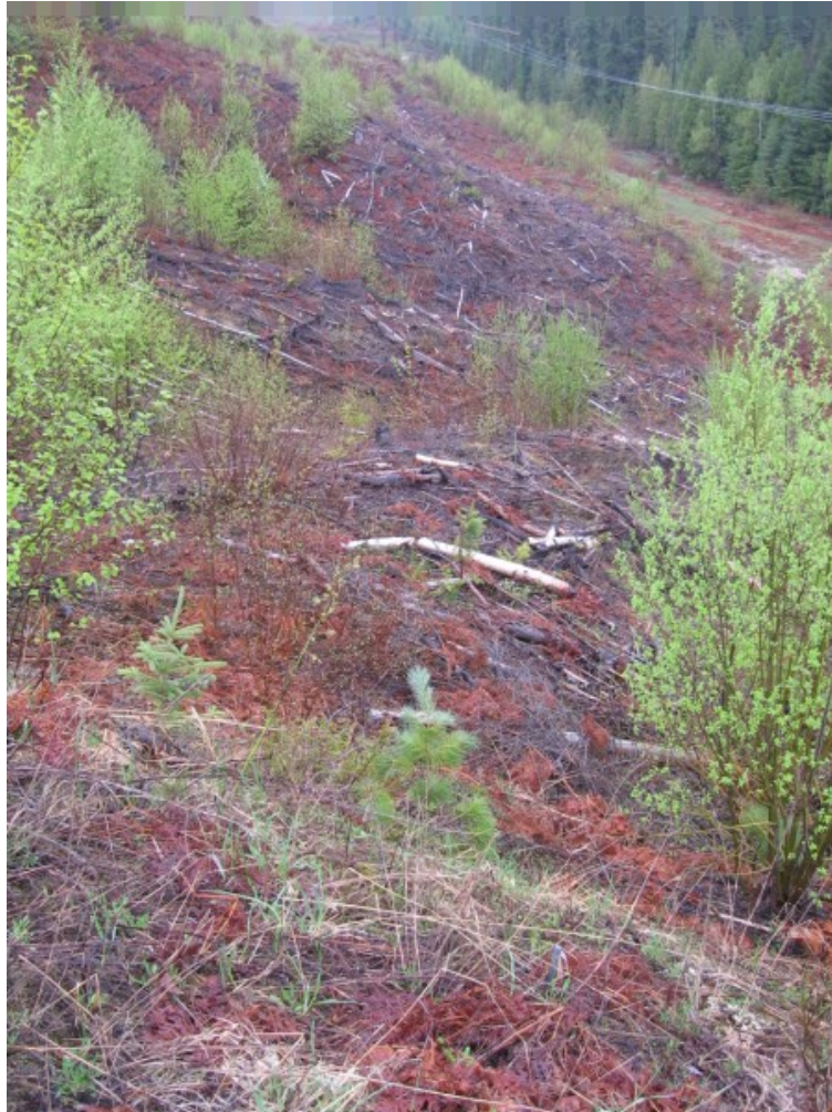
Figure 8. Debris created during vegetation clearing on transmission rights-of-way in Passmore.
