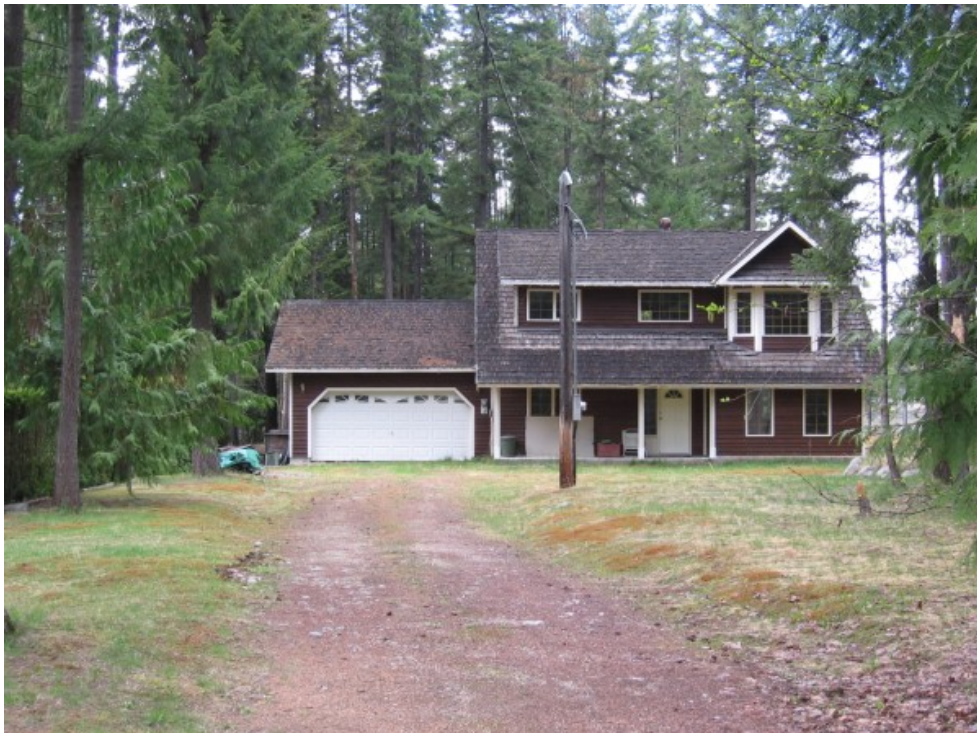
Figure 5. Example of Nakusp home with open decks and no setback to forest vegetation.
