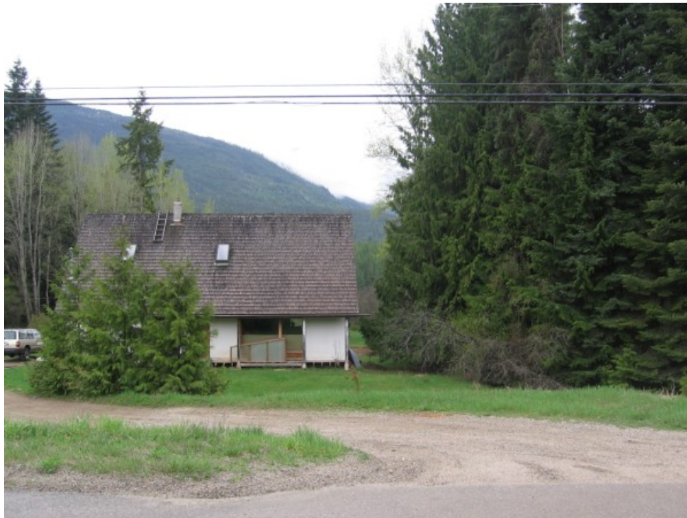
Figure 5. Home constructed with unrated roofing material and no setback from forest vegetation.
