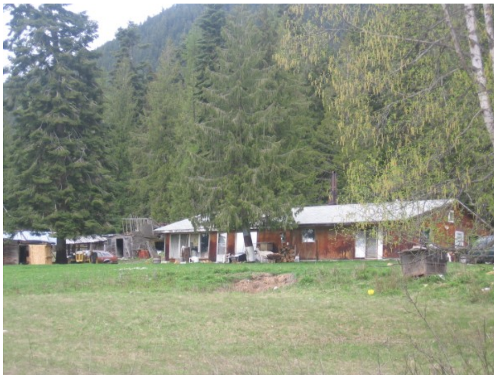
Figure 2. Photograph showing home with no setback to forest vegetation.
