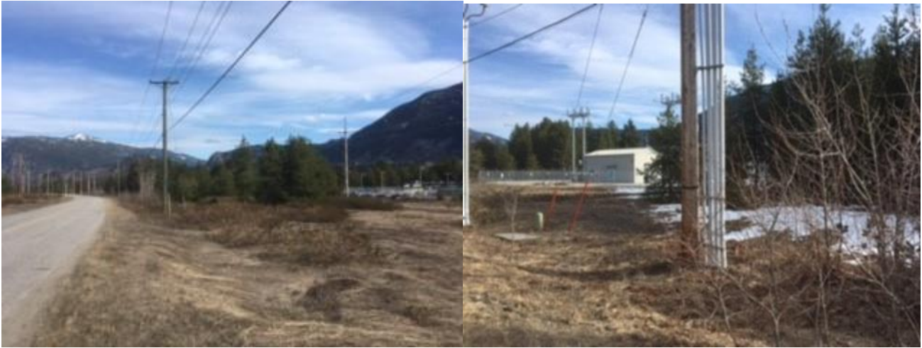
Figure 1: Facing North toward the electrical switching station
