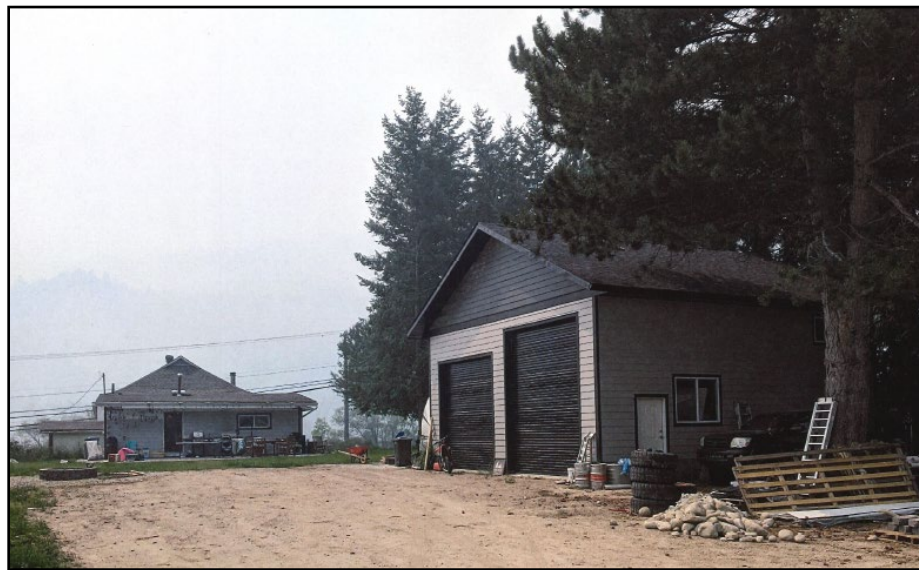
Figure 10: Photo of Existing Unauthorized Accessory Structure from Leckett Lane
