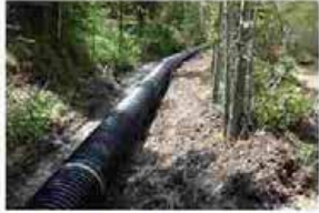
Boulder Creek Diversion Project
