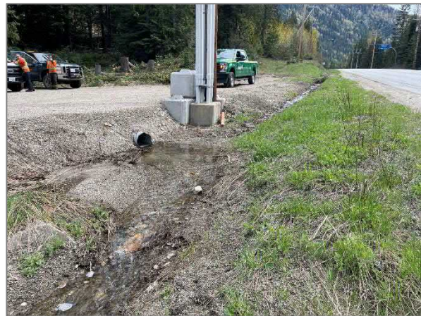
Photo 12. Ditch on the north side of Highway 6, supplying water to the property (May 10, 2023).
