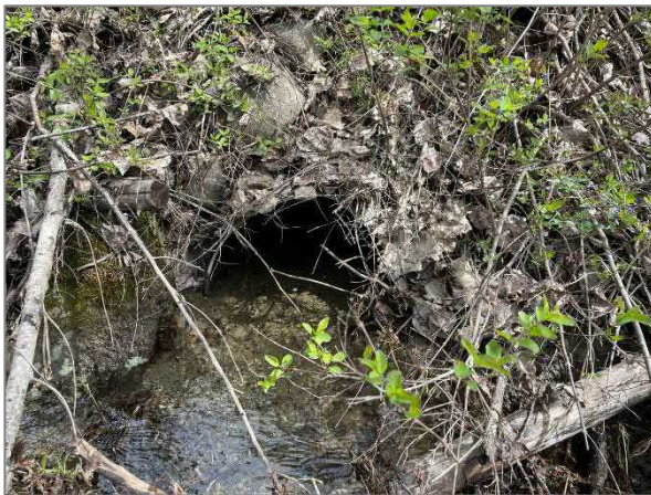
Photo 11. Water flow from culvert underneath highway 6 (May 10, 2023).
