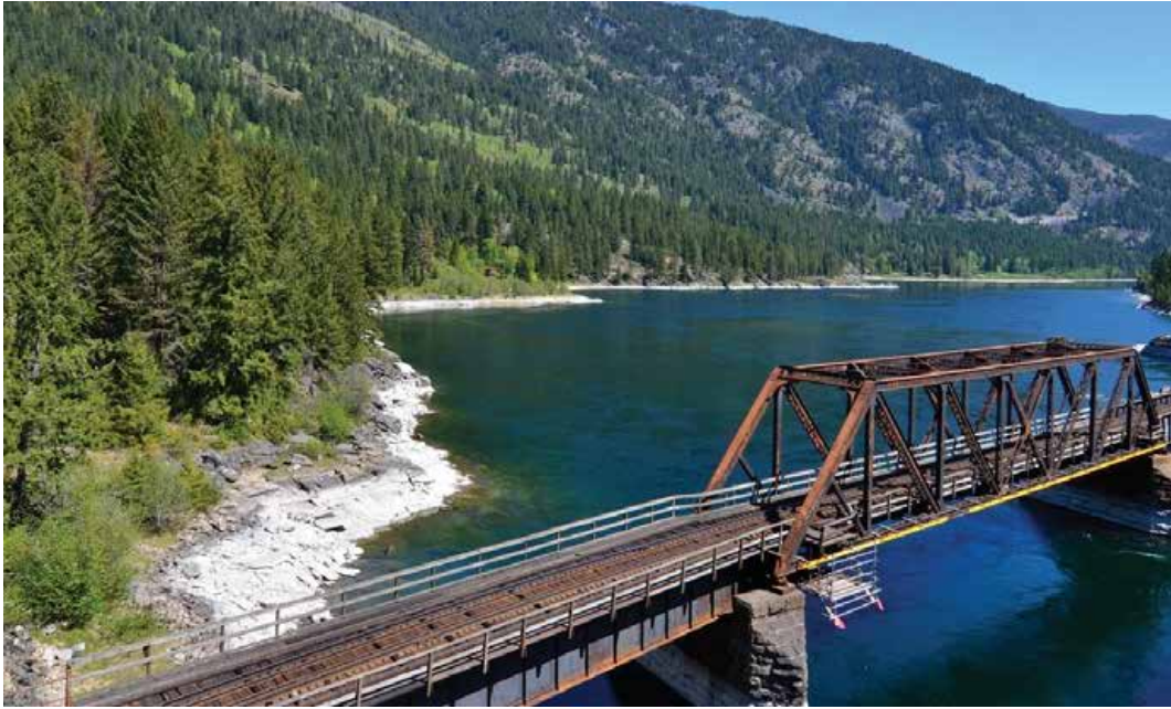
Figure 7. Railway bridge adjacent to Taghum Bridge. 25
