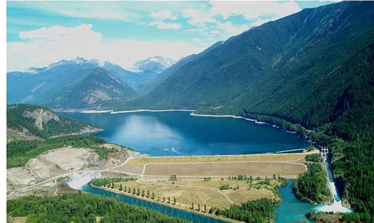
Figure 12. Duncan Dam, located south of Duncan Island on Duncan Lake 75
