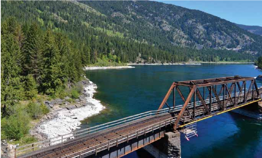
Figure 7. Railway bridge adjacent to Taghum Bridge. 25
