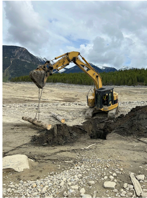
Bush Harbour temporary breakwater construction
