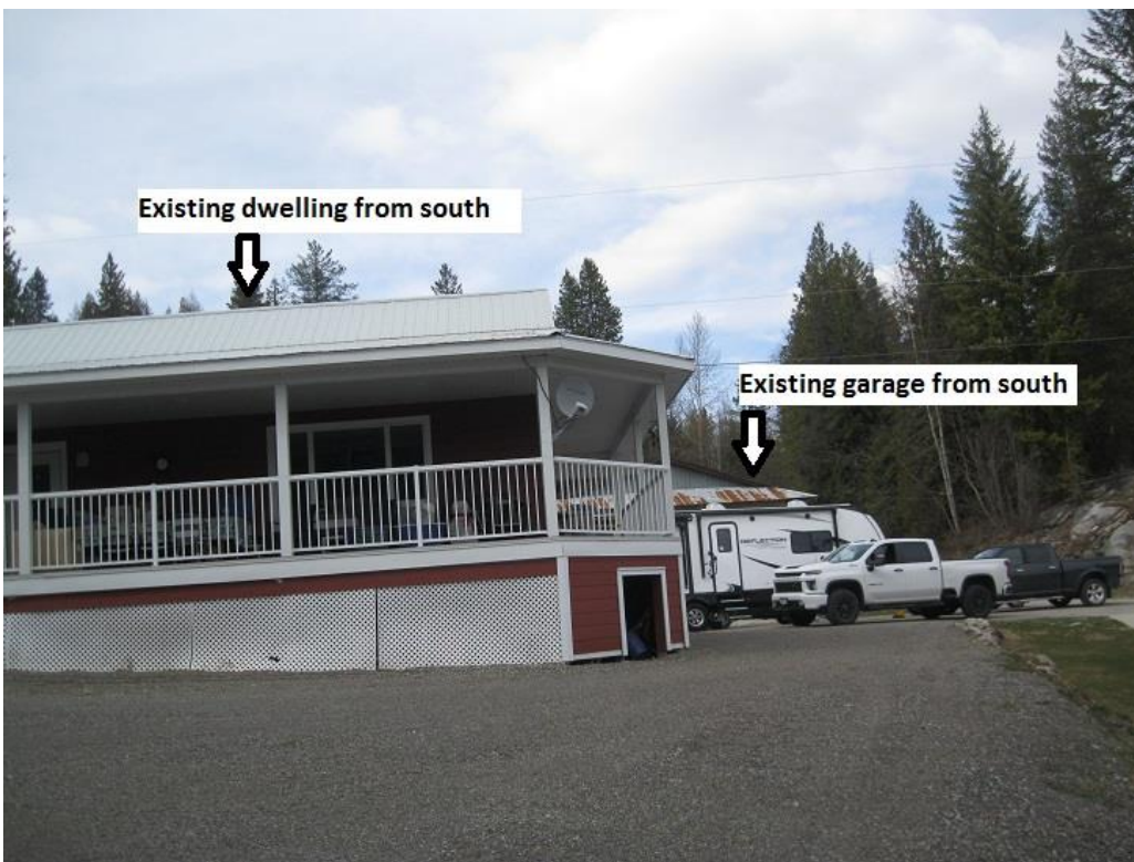
Figure 5; Facing North; both dwelling and garage visible in the image
