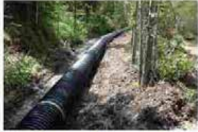
Boulder Creek Diversion Project
