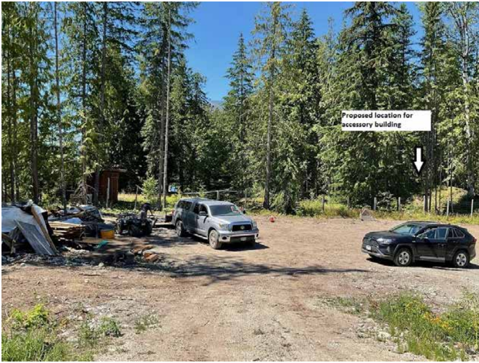
Figure 3: Area cleared and prepared for building
