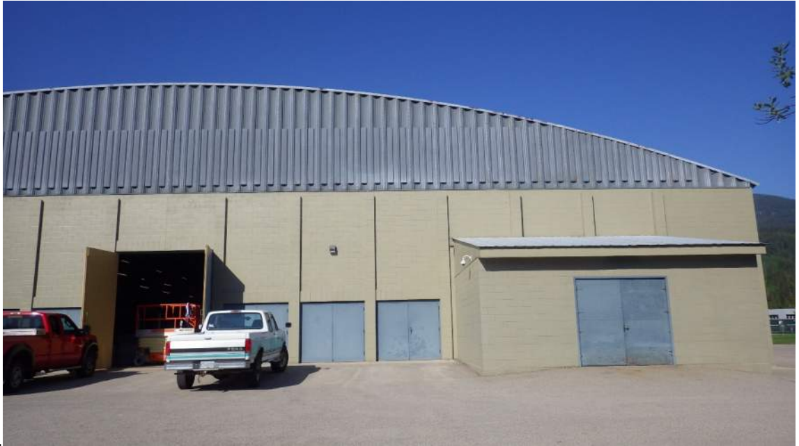
Typical gable end of roof.
