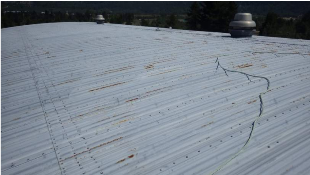
View of curved roofing panels with exhaust venting at the ridge.
