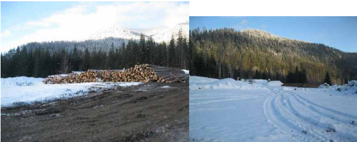
Figure 5: Log Yard Area Levelled to Date
