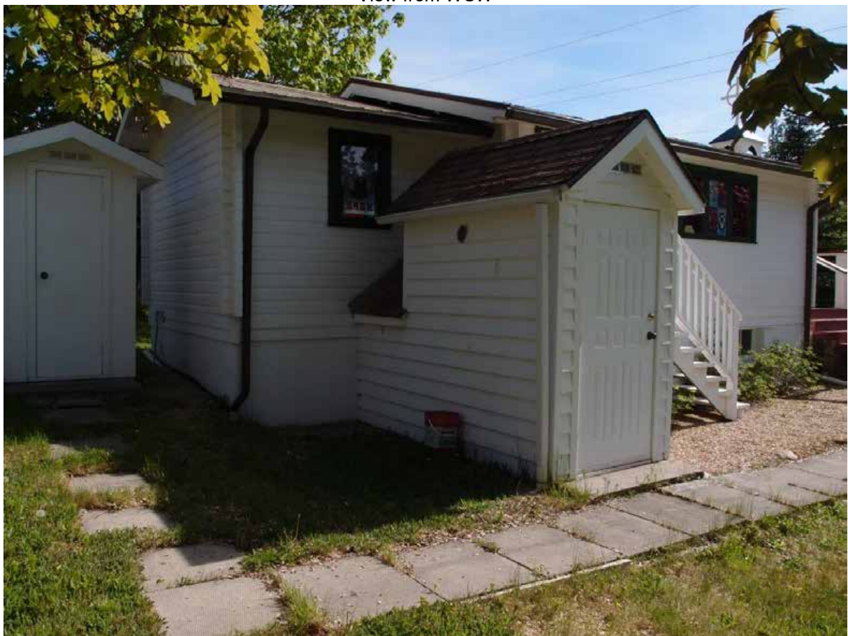
View from NNE; basement entry in foreground; pit toilet to left
