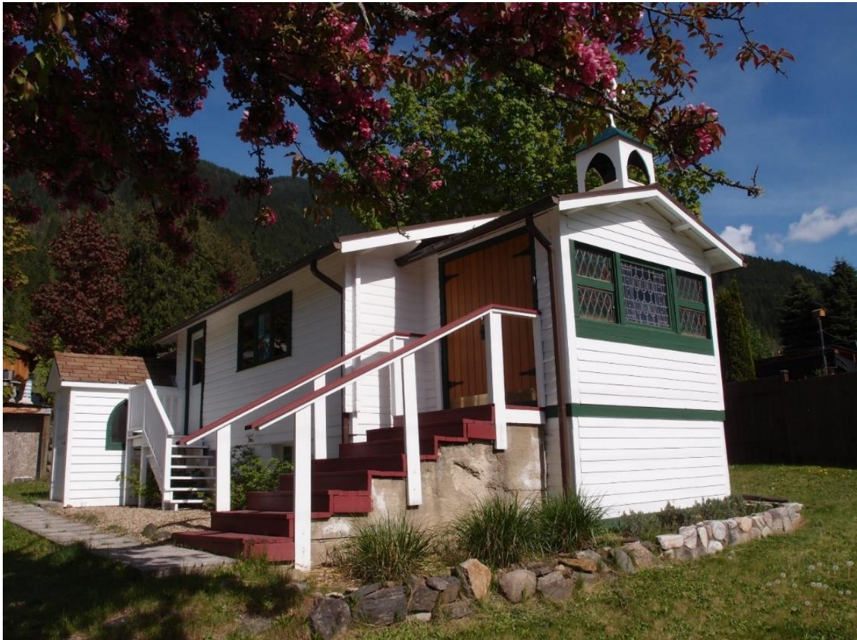
Closer view from NNW
