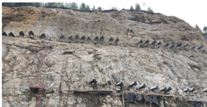
Installing protection for anchors.
