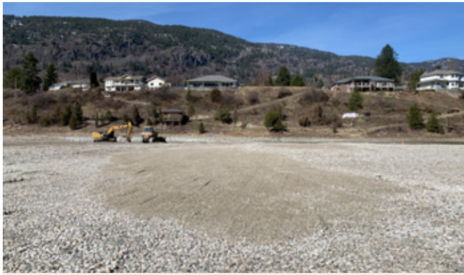
Recontouring in progress.
