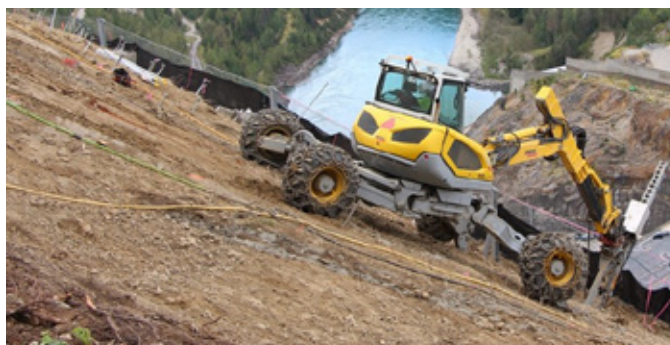
Tethered cat installing anchors.
