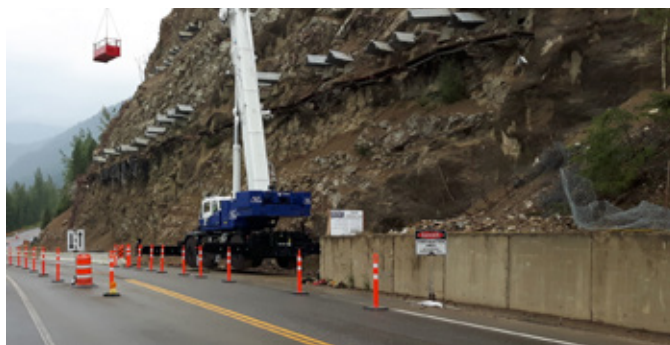
Crane being used to access the slope.
