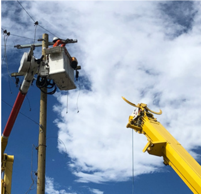
Crews work to replace a pole in Cranbrook in September 2020.
