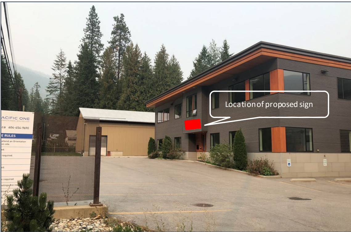
Figure 4: Front elevation of subject building, as seen from Lower Six Mile Rd
