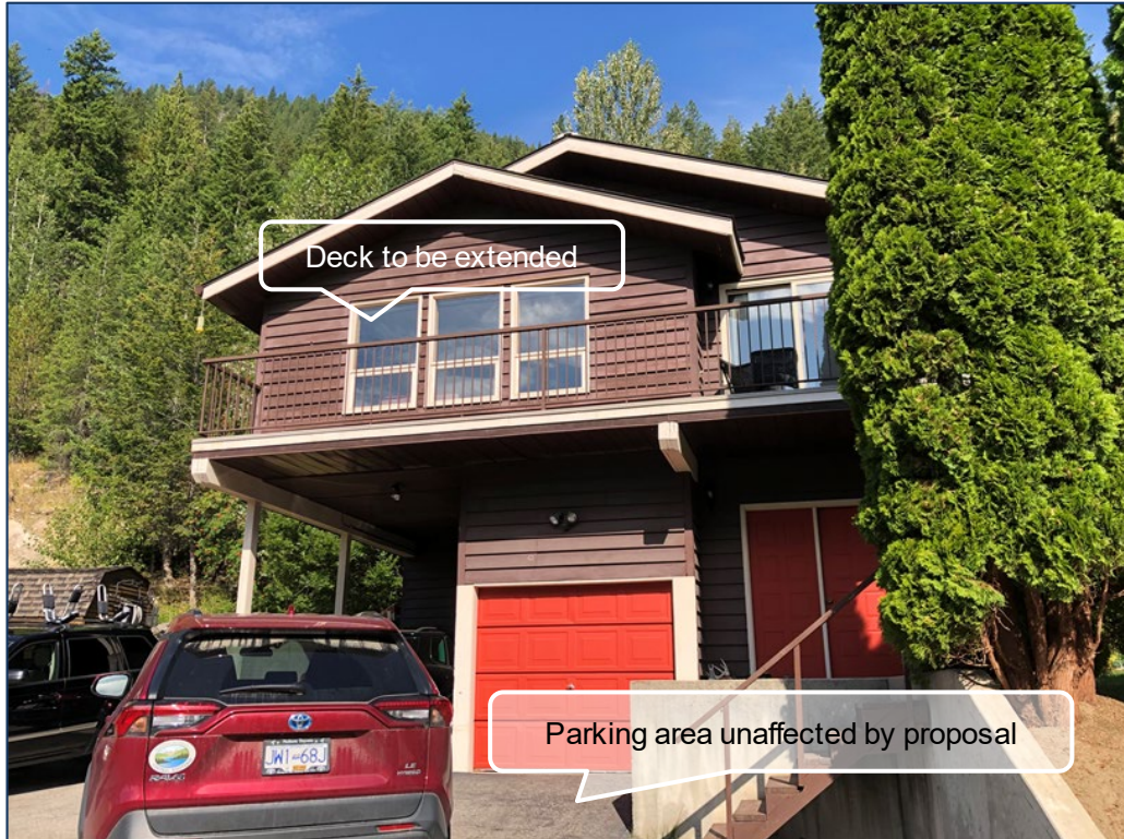
Figure 3: Front elevation of the dwelling showing the second floor deck which is proposed to be extended
