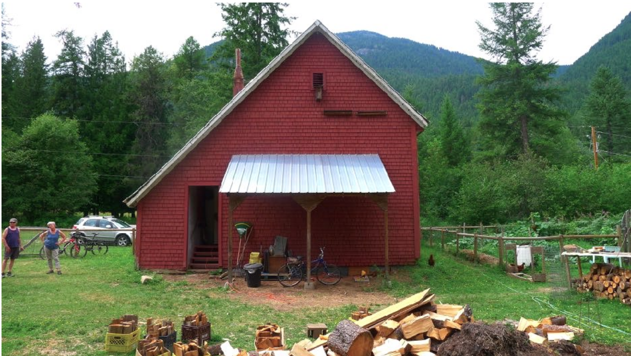
Top: Looking north east showing the lean-to extension, concrete chimney and its supports
