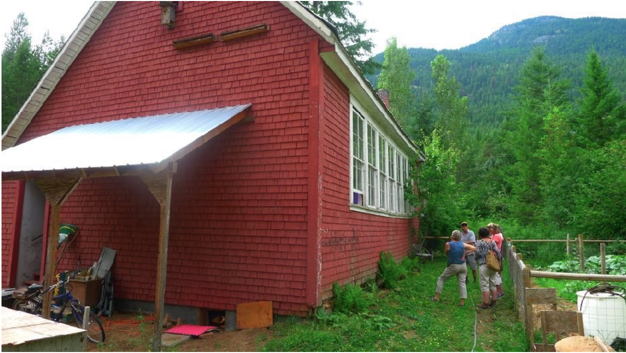
Rear and north side of the building
