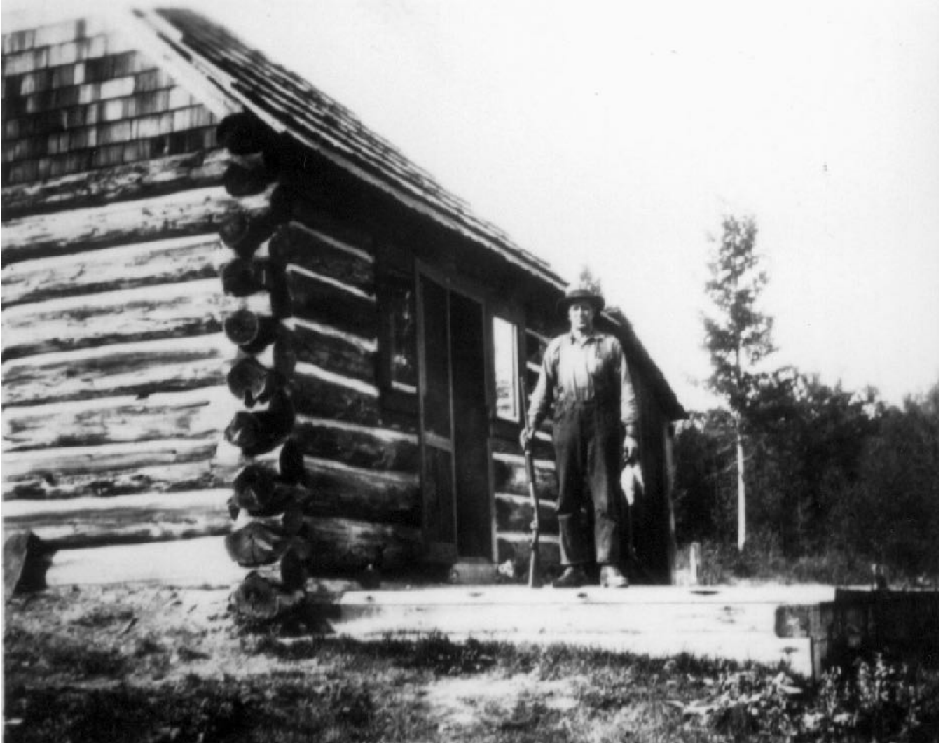
Above: Billy Clark at his cabin in the 1930s showing the door with side windows, shingled gable ends and shingled roof. Note the lack of fascia boards which were a later addition. source: BC Archives 193501-001
