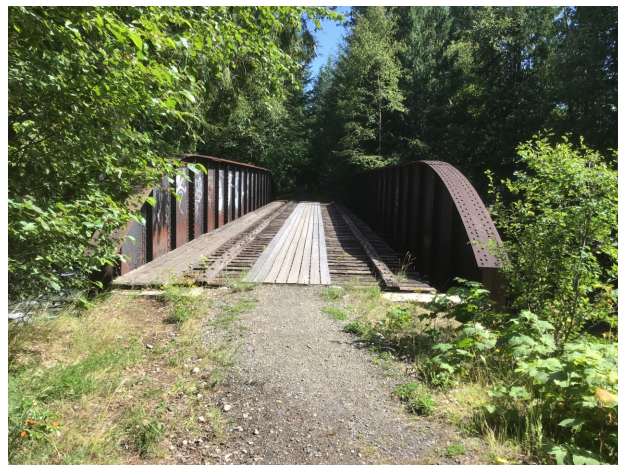
E) Nakusp and Slokan Railway Trail bridge deck.
