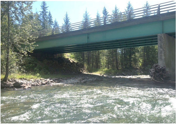
B) Mid channel, looking at left bank at rip rap armouring.
