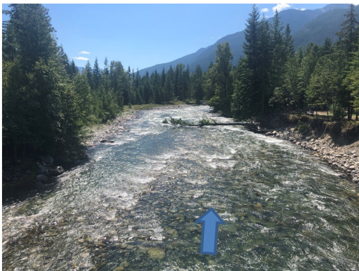
Photo 12. Looking downstream at Wilson Creek from on top of the Hwy 6 bridge. Photo: BGC, July 26, 2019.
