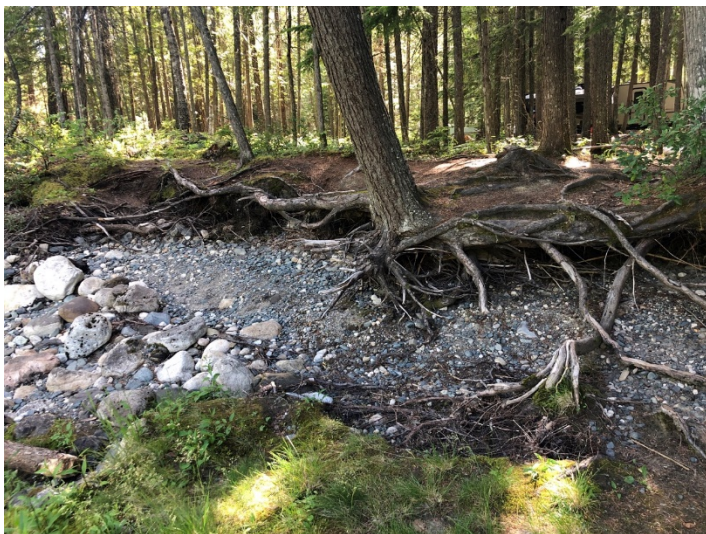
Photo 6. Standing on the edge of Wilson Creek, looking at erosion of the right bank along Roseberry Provincial Park, approximately 0.4 km upstream of the Highway 6 bridge. Photo: BGC, July 26, 2019.
