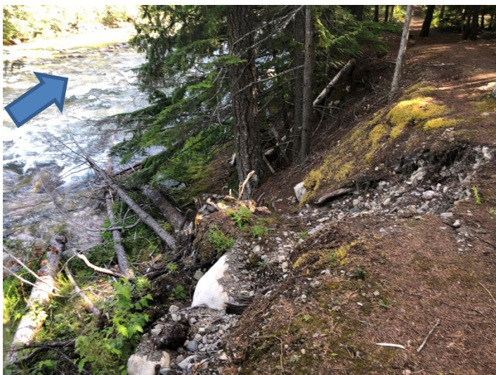
Photo 3. Standing on the right bank of Wilson Creek in Roseberry Provincial Park, approximately 0.5 km upstream of the Highway 6 bridge. Looking at erosion of the right bank. Photo: BGC, July 26, 2019.
