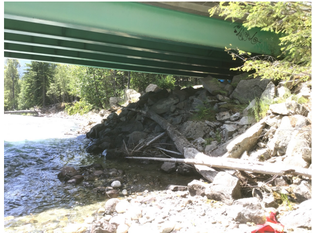
C) Looking downstream at right bank at rip rap armouring.
