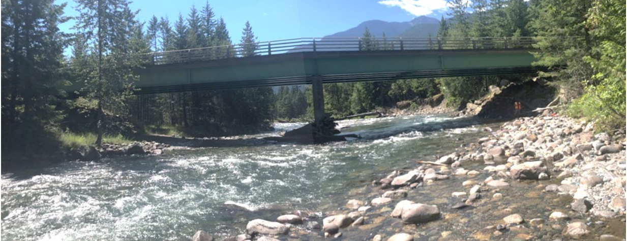
A) Looking downstream at Wilson Highway Bridge.
