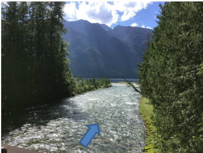
Photo 17. Standing on the rail bridge looking downstream at the Wilson Creek outlet to Slocan Lake. Note mid-channel cobble deposit. Photo: BGC, July 26, 2019.
