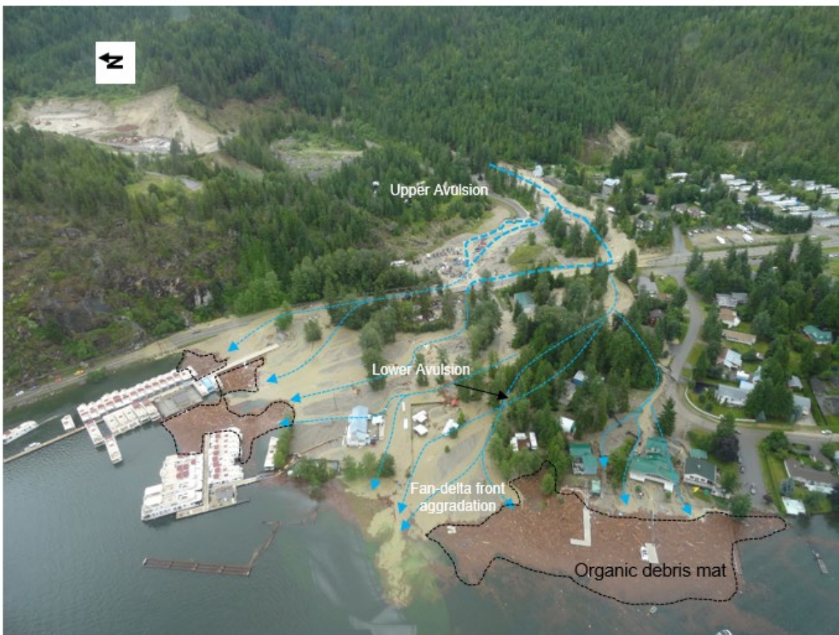
Figure 2-7. Debris flood on Sicamous Creek, on Mara Lake, British Columbia, on June 24, 2012 showing widespread avulsions indicated by blue arrows and leading to multi-million dollar losses and legal action. A lower and upper avulsion occurred, one on the distal portion of the delta and one upstream of the highway bridge. Both united to inundate the topographically lower northern portion of the fan.
