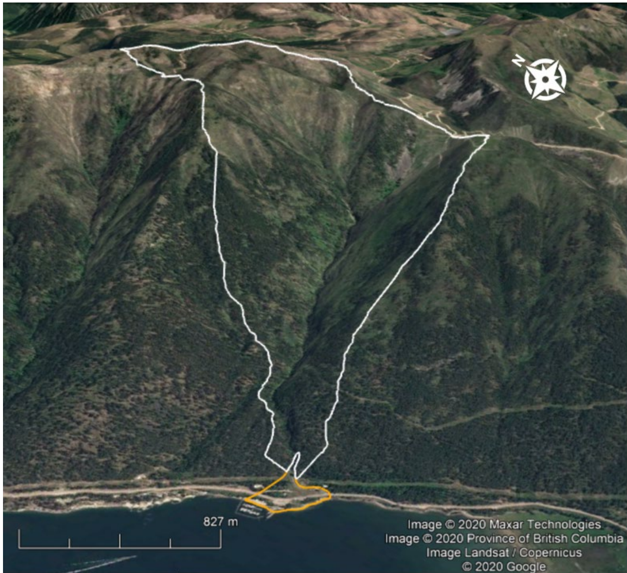
Figure 1-2. A Google Earth image of a typical steep creek, a debris-flow prone watershed (Kuskonook Creek) located north of Creston in the RDCK. The approximate watershed and fan boundary are outlined in white and orange, respectively.
