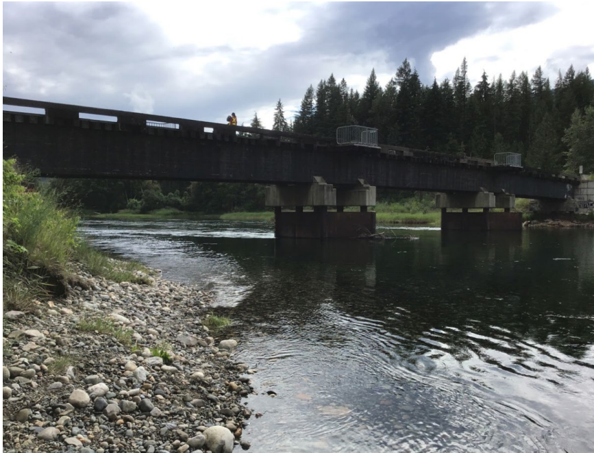
Photo 5. From left bank looking downstream at Logging Bridge. Photo: BGC, July 2, 2019.
