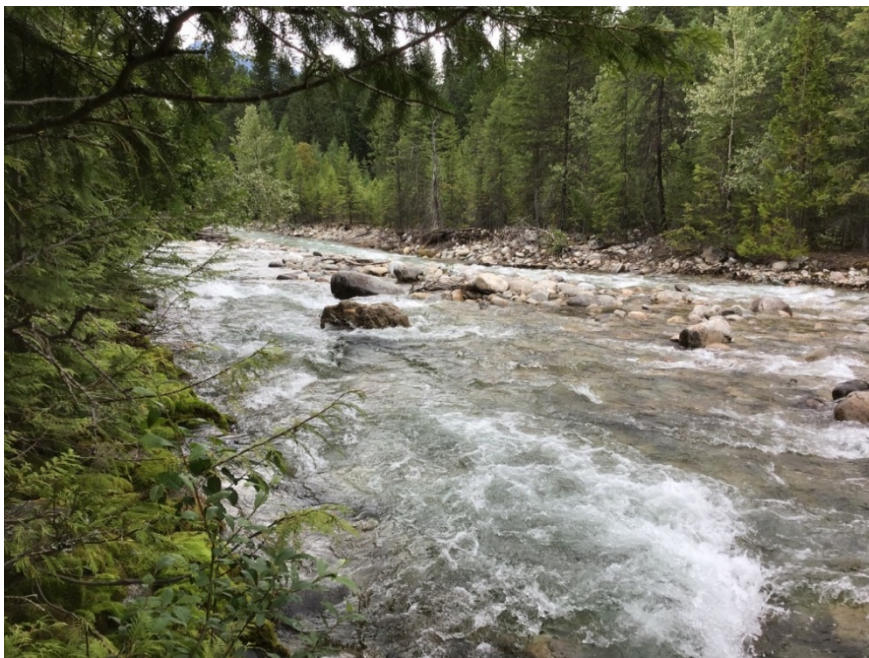
Photo 14. Lemon Creek rock protection on left bank 200 m west of Highway 6. Photo: BGC, July 2, 2019.
