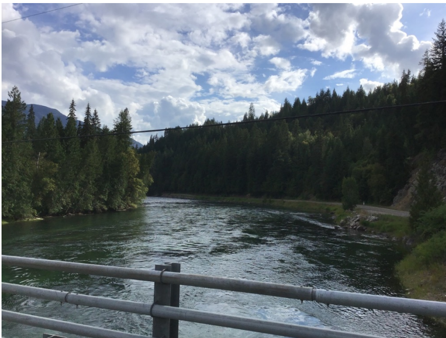
Photo 24. Standing on Winlaw Bridge looking downstream. Photo: BGC, July 2, 2019.
