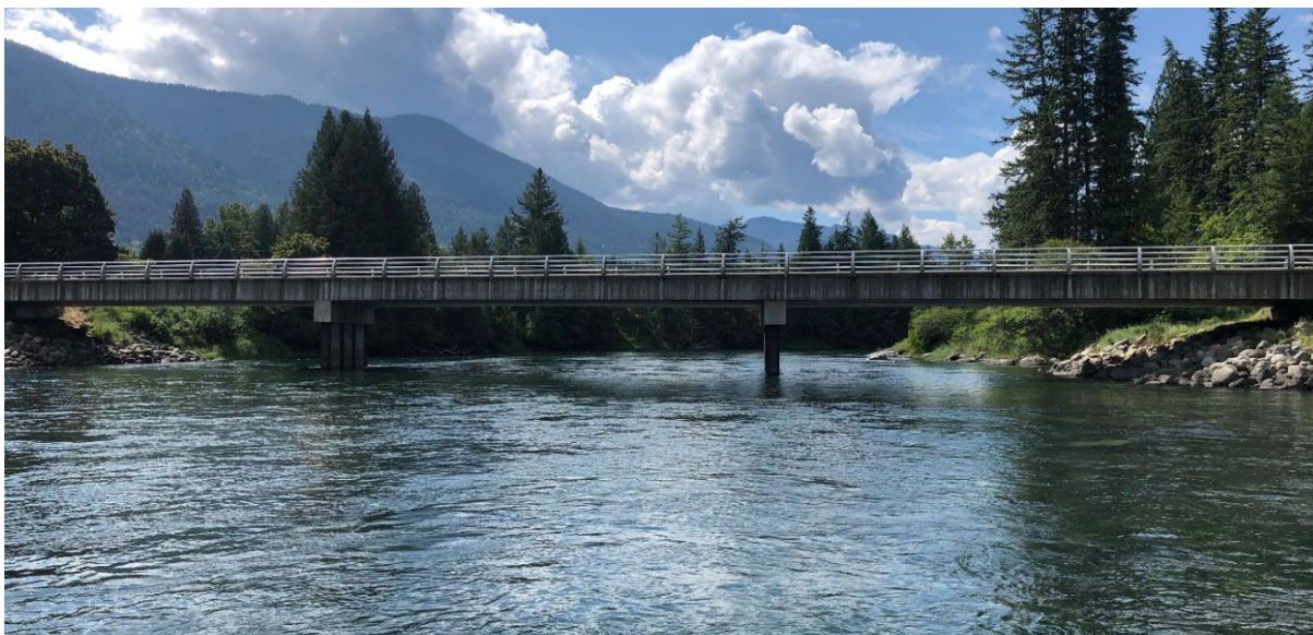
Figure E-7. Slocan City Bridge over the Slocan River looking downstream. Photo: Midwest Survey July 8, 2019.
