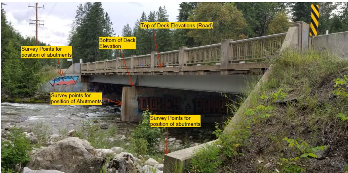
Figure 4-2. Example of bridge structure features collected during the Slocan River survey.
