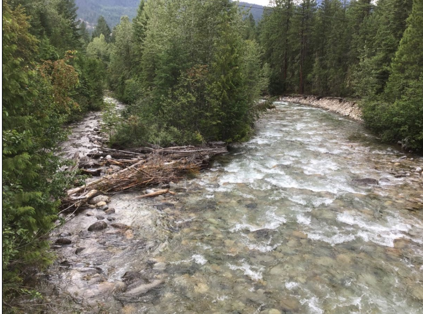
Photo 17. From Highway 6 Bridge over Lemon Creek looking downstream. Photo: BGC, July 2, 2019.
