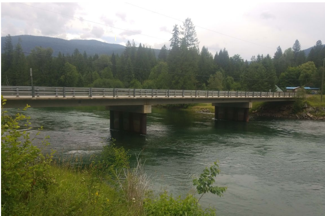
Figure E-18. Winlaw Bridge over the Slocan River looking upstream from the right bank. Photo: Midwest Survey July 7, 2019.
