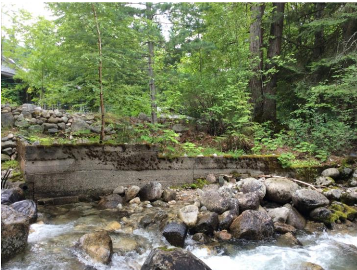
Photo 11. On right bank looking at left bank low wall constructed of rounded cobbles, approximately 30 m downstream of the Hwy 3A bridge. Photo: BGC, July 4, 2019.
