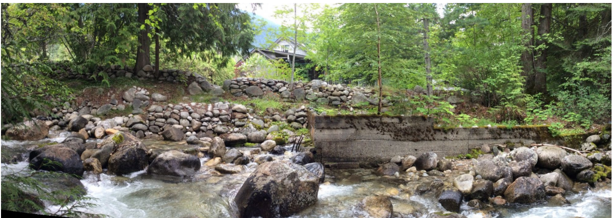
B) Berm constructed of rounded cobbles and old concrete foundation approximately 2 m high on left bank approximately 20 m downstream of Highway 3A bridge (STK-FP-4).
