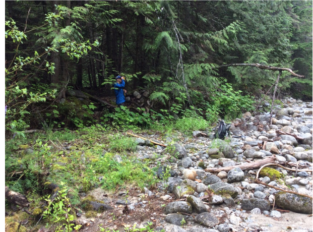
C) Low point in berm (STK-FP-6) on right bank approximately 275 m downstream of Hwy 3A. Right bank berm height was 0.6 m, left bank was 0.7 m compared with 1.2 m high upstream and downstream of this location on both banks.
