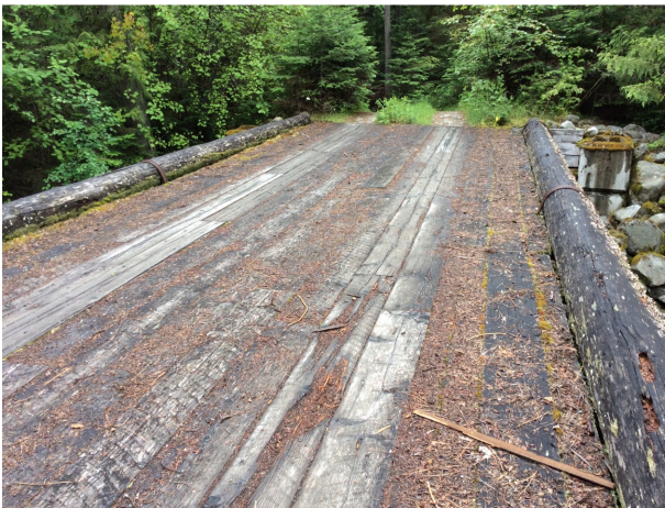
E) Wooden trestle bridge
