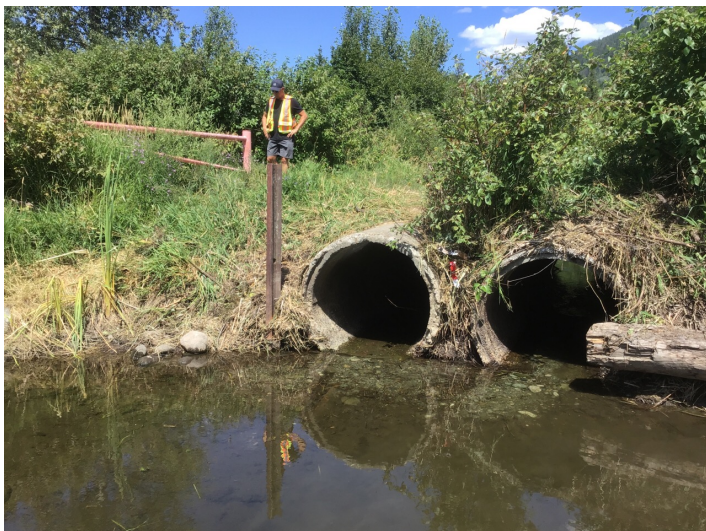
Photo 6. Culverts from Erie Lake emptying into Erie Creek. Photo: BGC, July 31, 2019.
