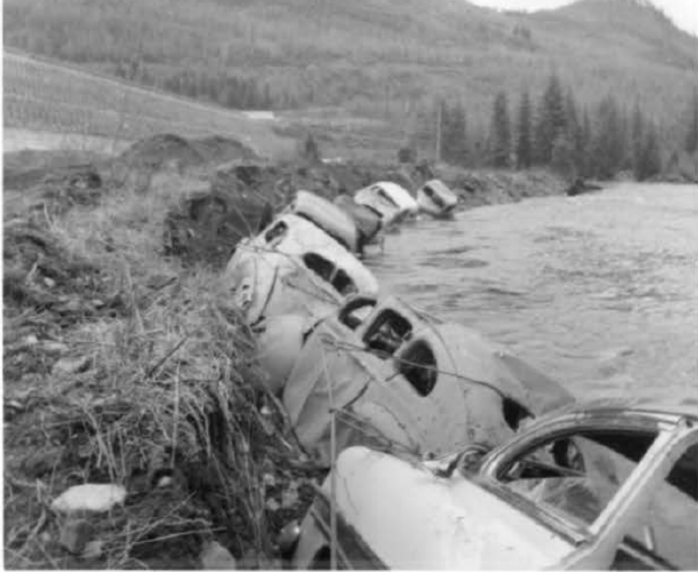
Figure 3-5. “Junk” car bodies placed along the CanEx tailings disposal area. Looking downstream. Photo: CanEx (1963).
