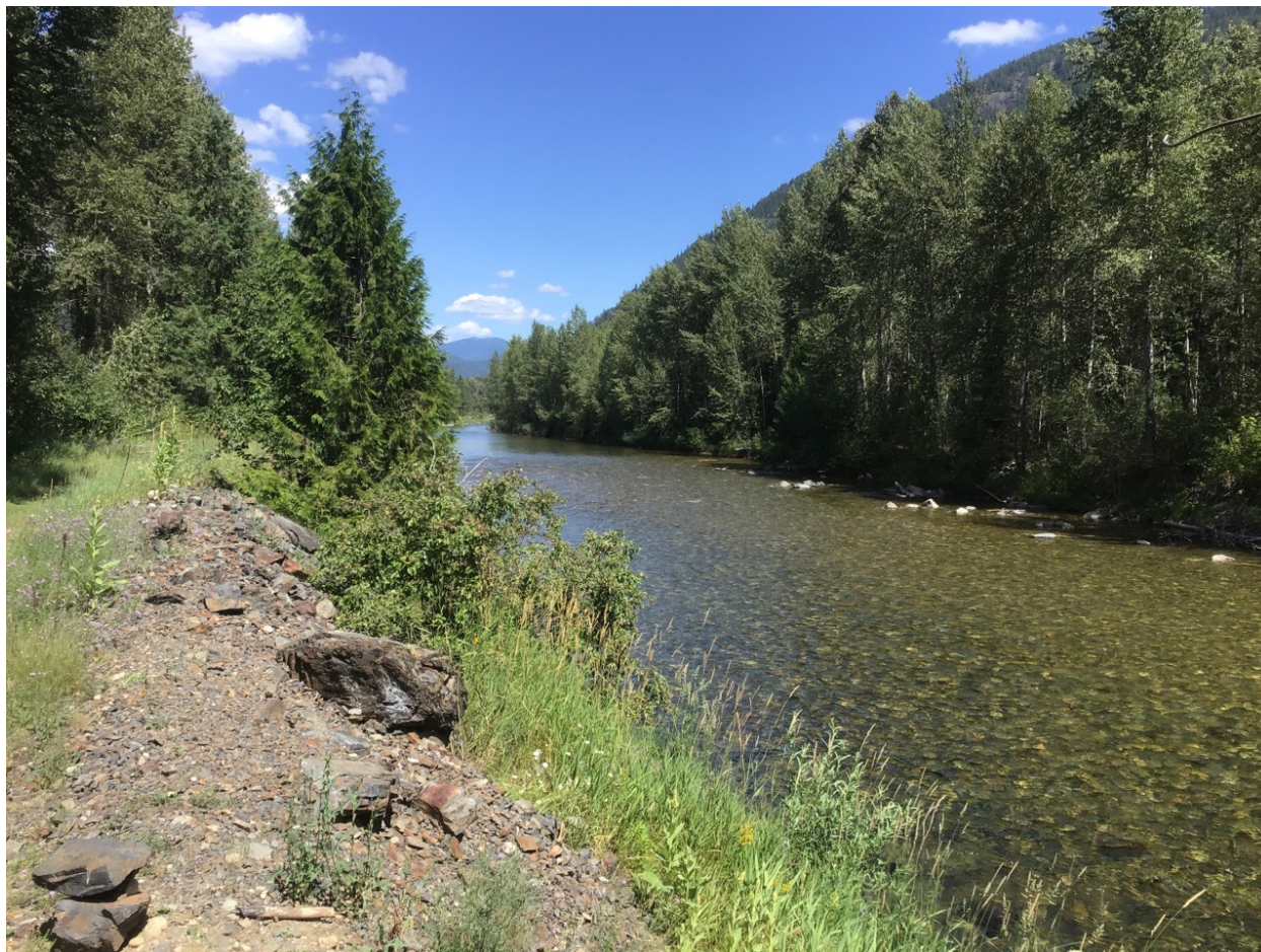
Figure 3-4. Dike on the right bank of the Salmo River, looking upstream towards the Village of Salmo. Photo: BGC, July 31, 2019.
