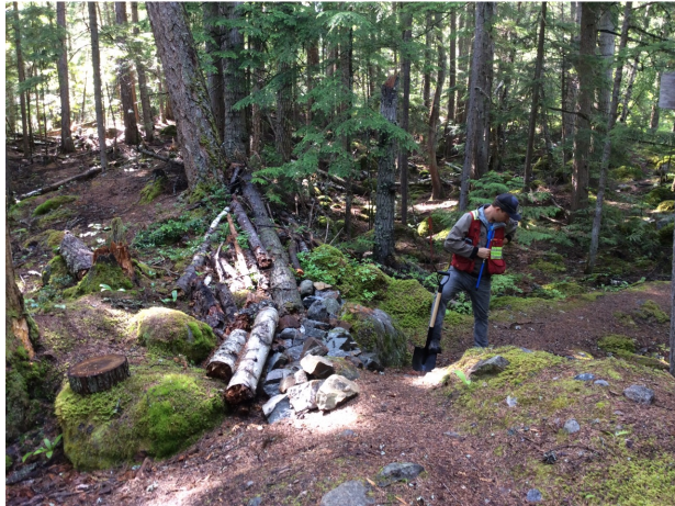
RFS-LP-01. On the right bank looking southeast at low point (i.e., walking trail) in natural berm.
