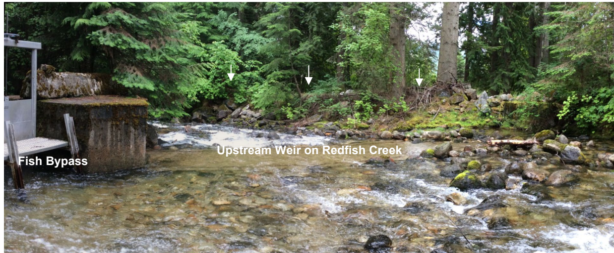
Looking downstream (south) at upstream weir on Redfish Creek with fish bypass to the left, and dike on right bank (RFS-FP-01). Arrows indicate dike crest.
