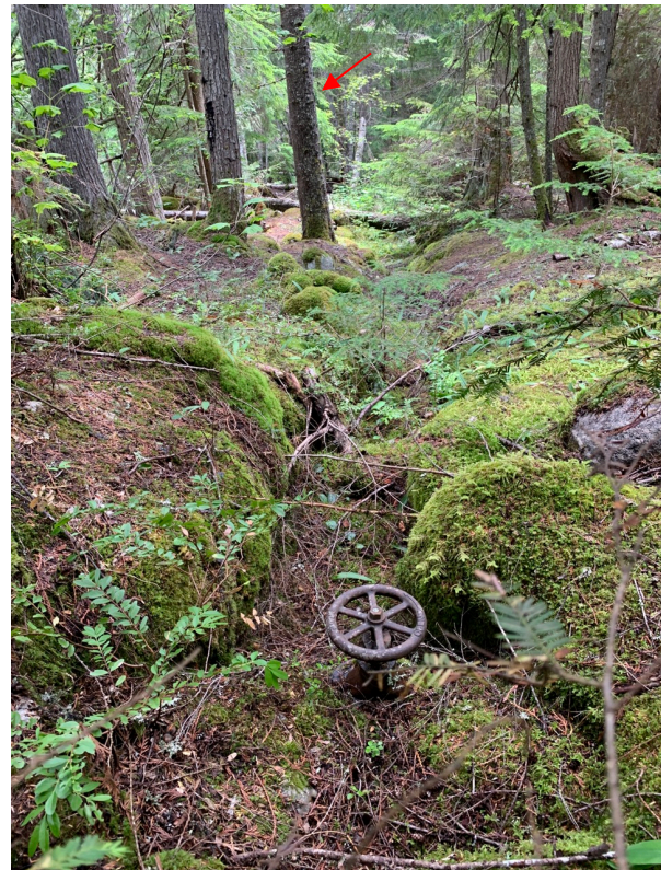
RFS-LP-02. Looking south valve of water intake and along pipe trench (pipe removed). For reference, note arrow indicating same tree as in image above.
