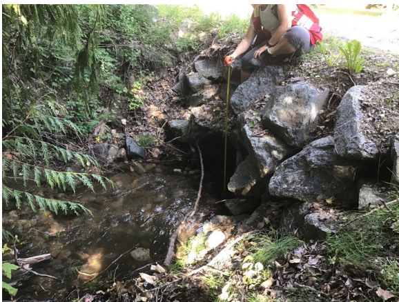
E) PRT-CV-5. Looking at outflow of Jones Road culvert
