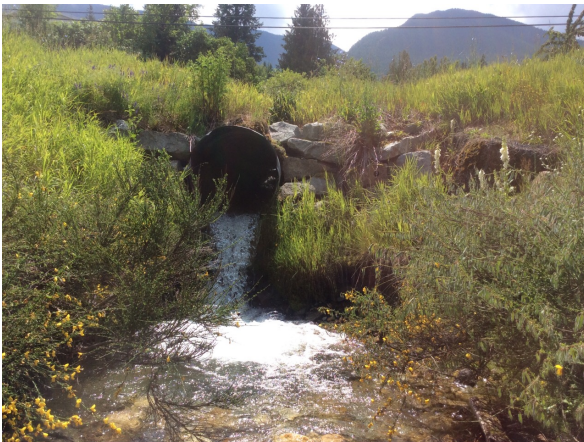
C) PRT-CV-3. Looking upstream at the outlet of Railway Avenue culvert.
