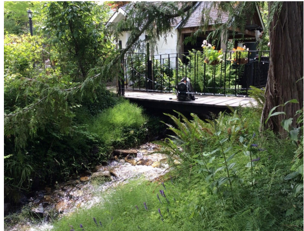
D) PRT-BR-4. Wooden footbridge with metal railing approximately 5 m wide, 1.6 m high.
