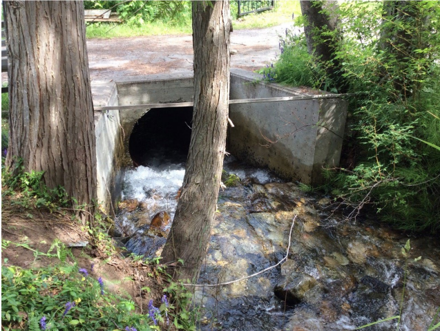
A) PRT-CV-1. Looking upstream towards the culvert at Woodside Avenue.
