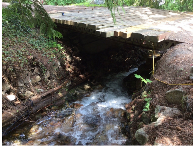
B) PRT-BR-2. Looking downstream towards a wooden bridge with metal frame.
