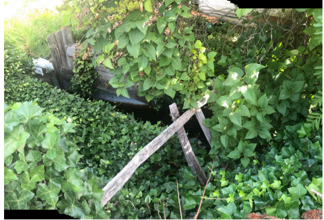
B) Metal flashing containing the creek upstream of Procter Lane
