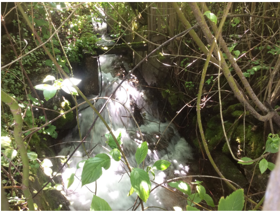
C) Looking upstream of Railway Avenue at concrete flume.
