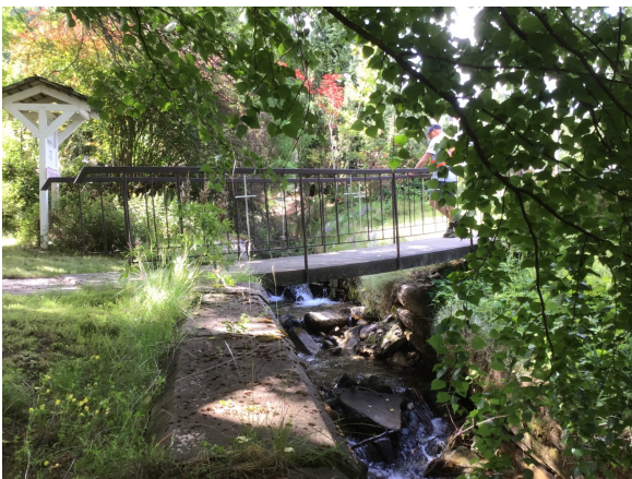
E) PRT-BR-5. On right bank looking upstream at church bridge.
