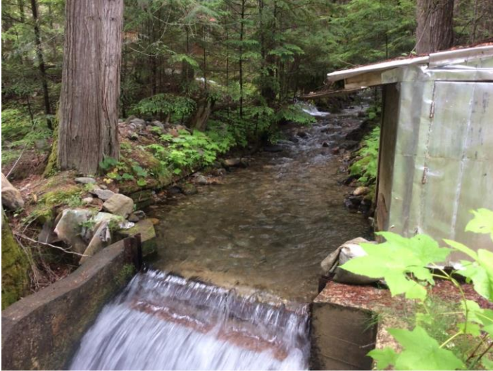
Photo 9. Looking upstream (south) at the water intake on Procter Creek. Photo: BGC, July 6, 2019.
